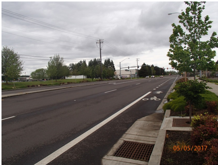
Figure 1: DFI No. D00707, looking West
