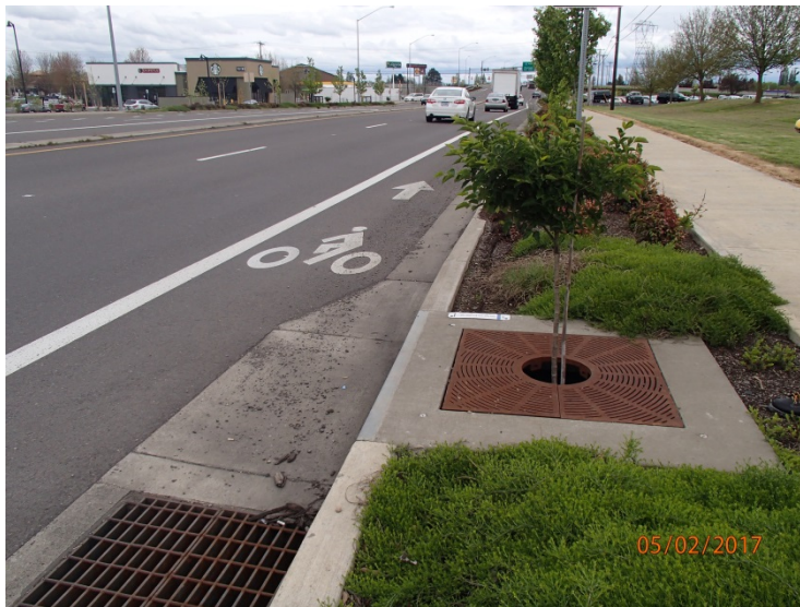
Figure 1: DFI No. D00706, looking East
