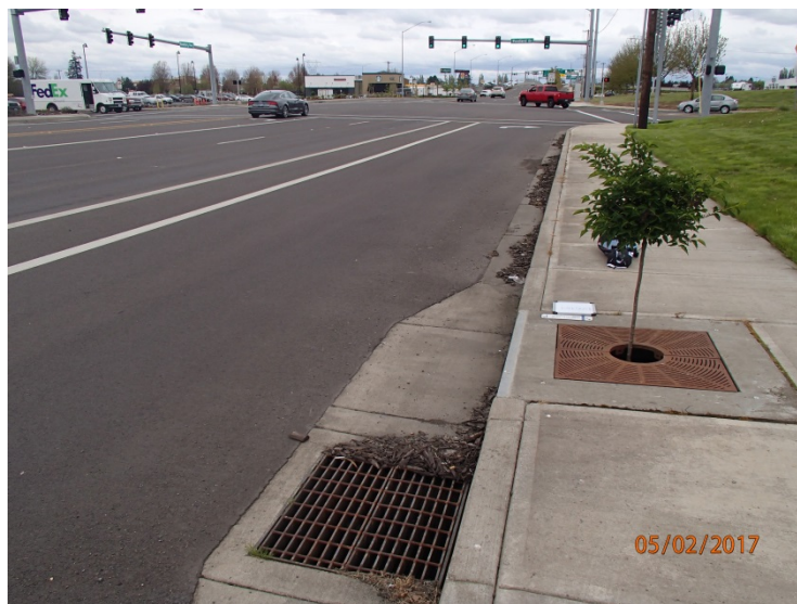
Figure 1: DFI No. D00704, looking East
