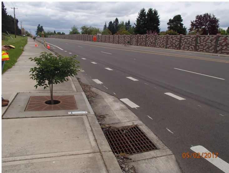
Figure 1: DFI No. D00700, looking West
