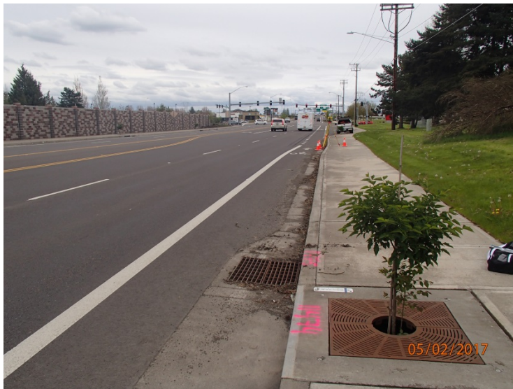
Figure 1: DFI No. D00698, looking East
