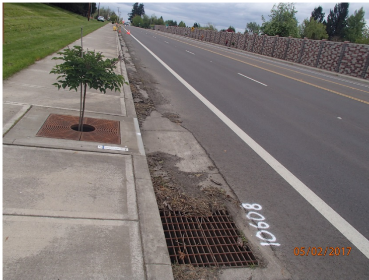
Figure 1: DFI No. D00696, looking West
