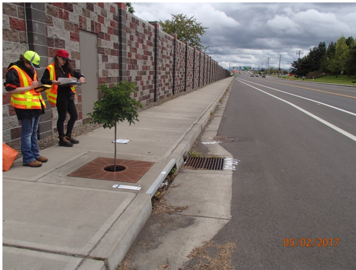
Figure 1: DFI No. D00693, looking East
