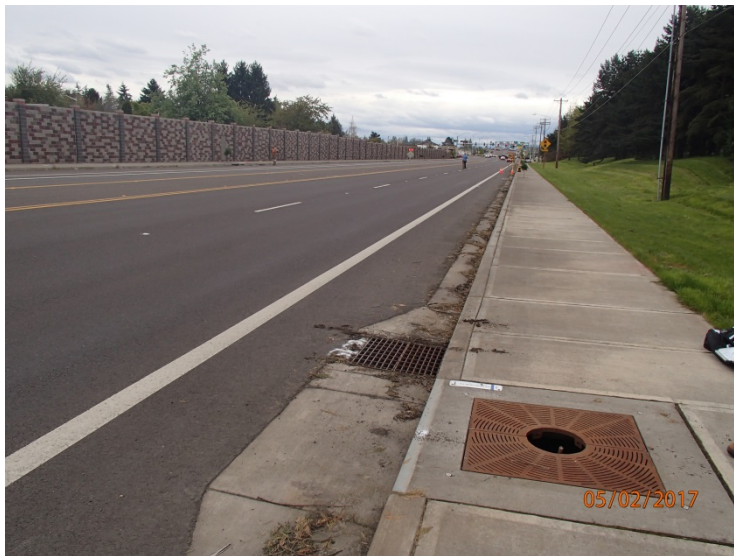
Figure 1: DFI No. D00692, looking East
