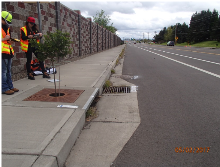
Figure 1: DFI No. D00691, looking East
