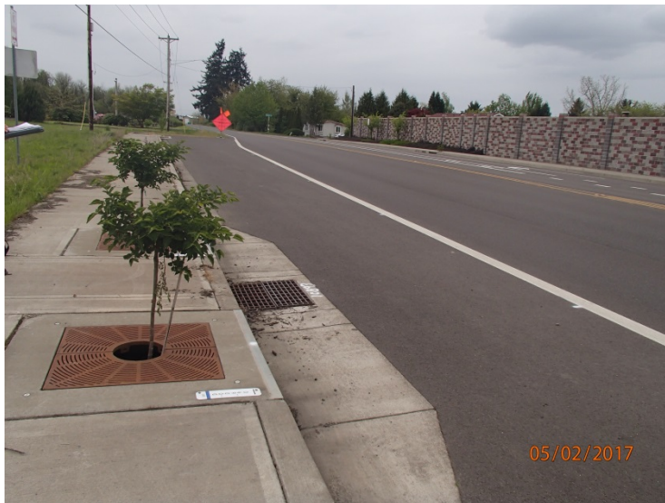
Figure 1: DFI No. D00690, looking West
