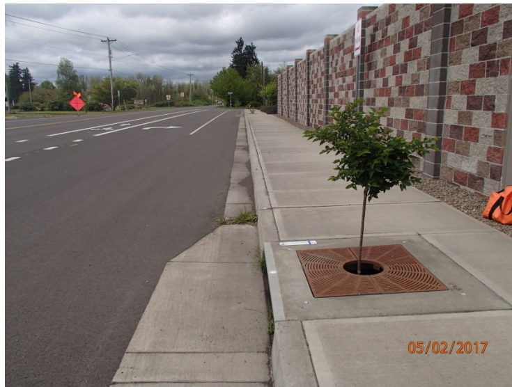
Figure 1: DFI No. D00687, looking West
