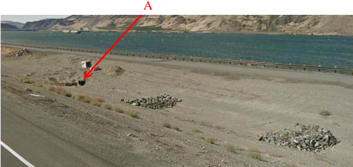
Figure 1 – Biofiltration Swale Outlet
