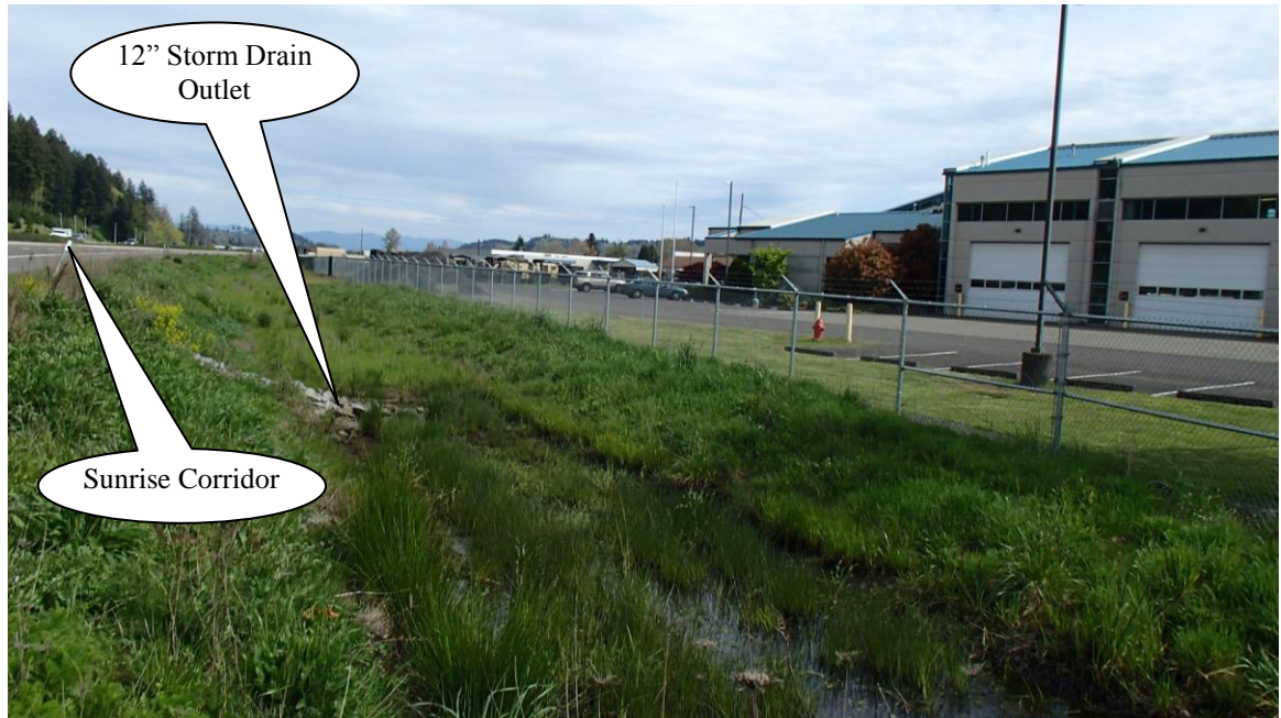
Photo 1: a view of water quality swale, looking Southeast.
