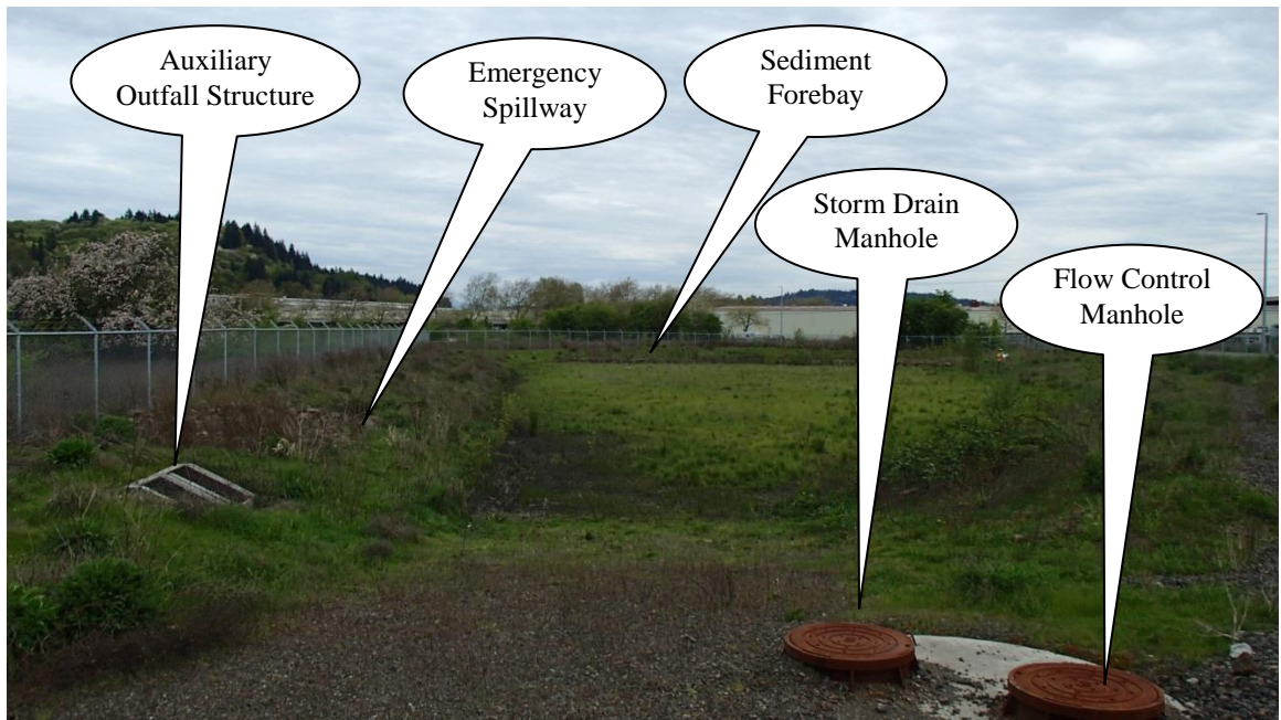
Photo 2: a view of extended detention pond, looking Southeast.
