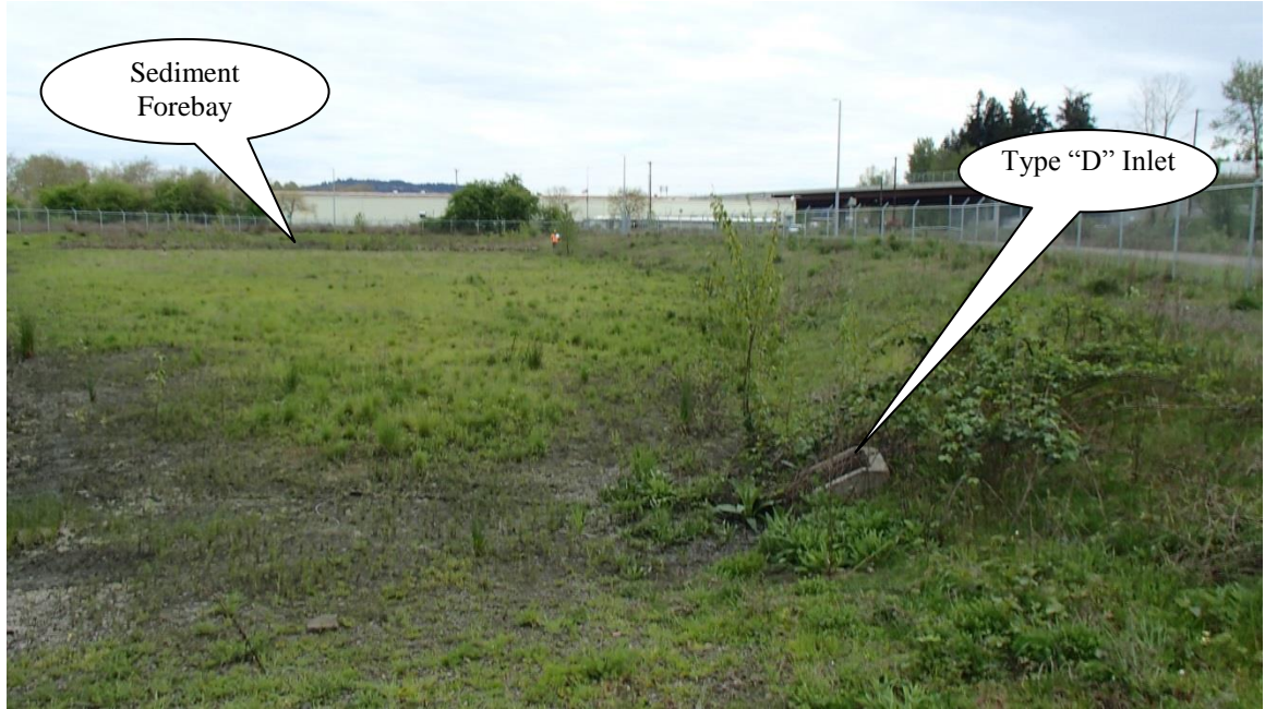
Photo 1: a view of extended detention pond, looking Southeast.
