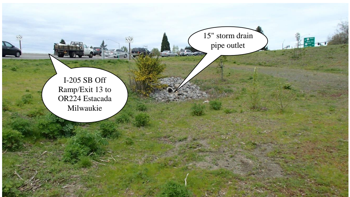
Photo 2: a view of bio-retention pond, looking Northeast at storm drain pipe outlet.
