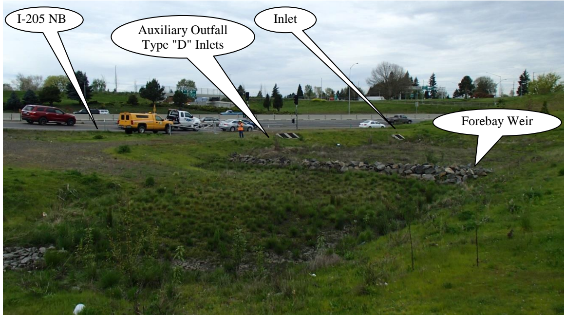
Photo 1: a view of bio-retention pond facility looking Northwest toward I-205 NB.
