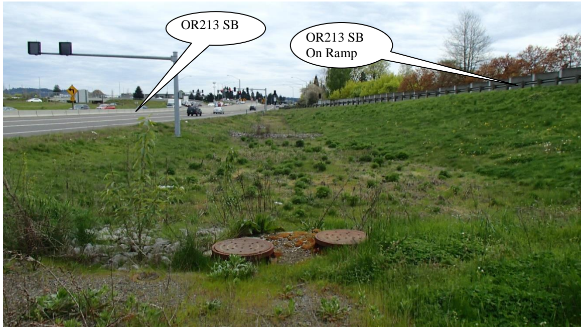
Photo 1: a view of storm drain and flow control manholes, looking South along OR213.
