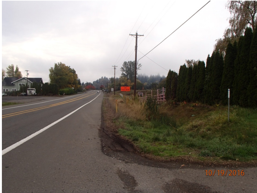
Figure 3: Right highway shoulder on Wallace Rd NW heading south
