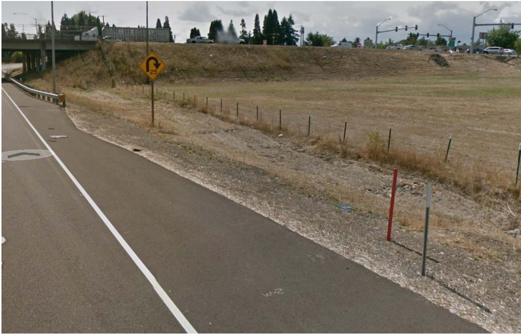
Figure 3: Access via roadside shoulder
