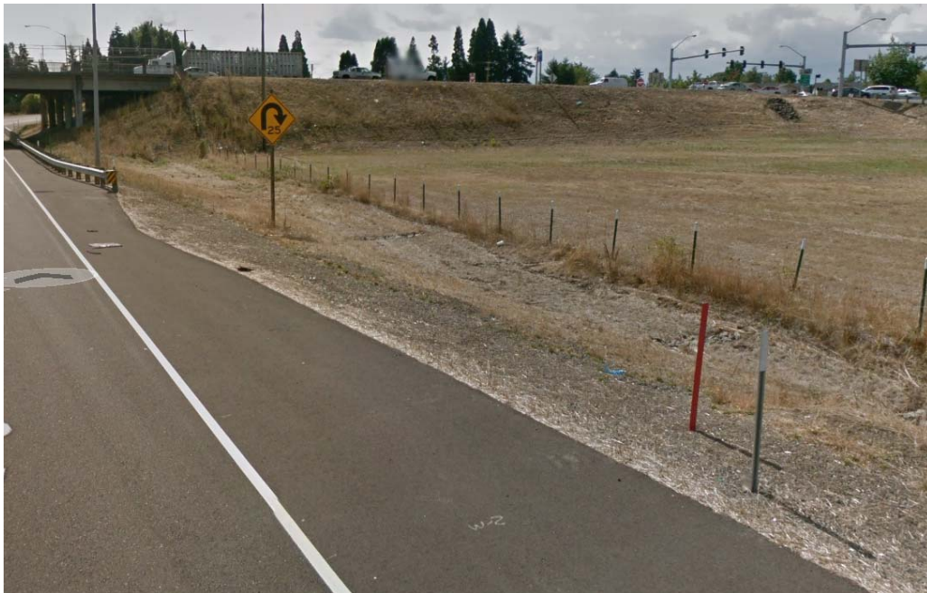
Figure 1: DFI No. D00645, looking South
