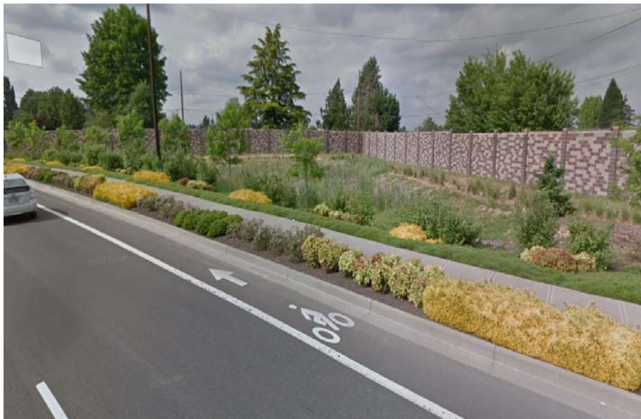
Figure 1: DFI No. D00644, looking North on WB Hillsboro-Silverton Hwy
