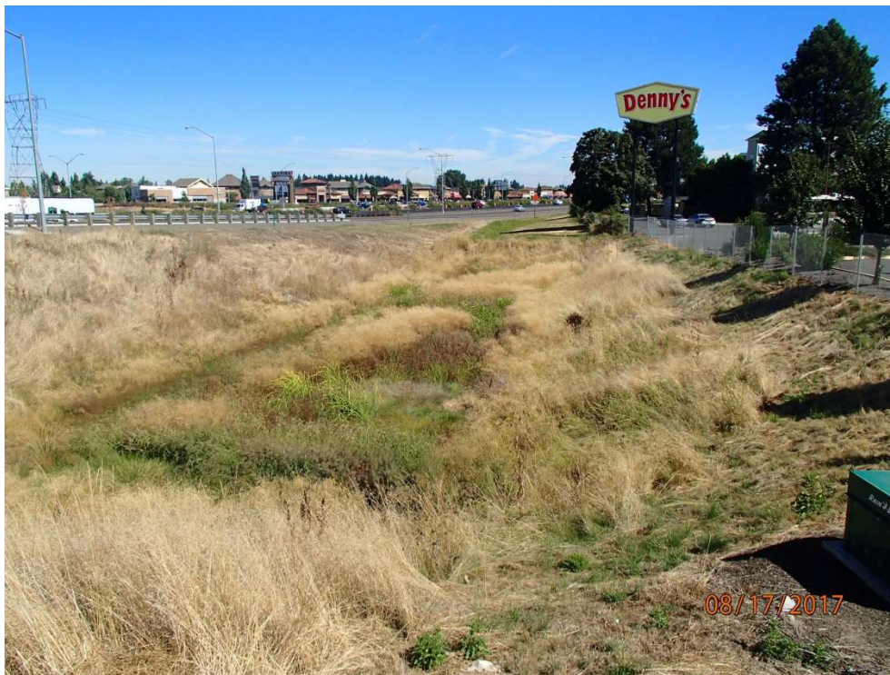
Figure 1: Detention Pond / Water Quality Biofiltration Swale Combo (D00643)
