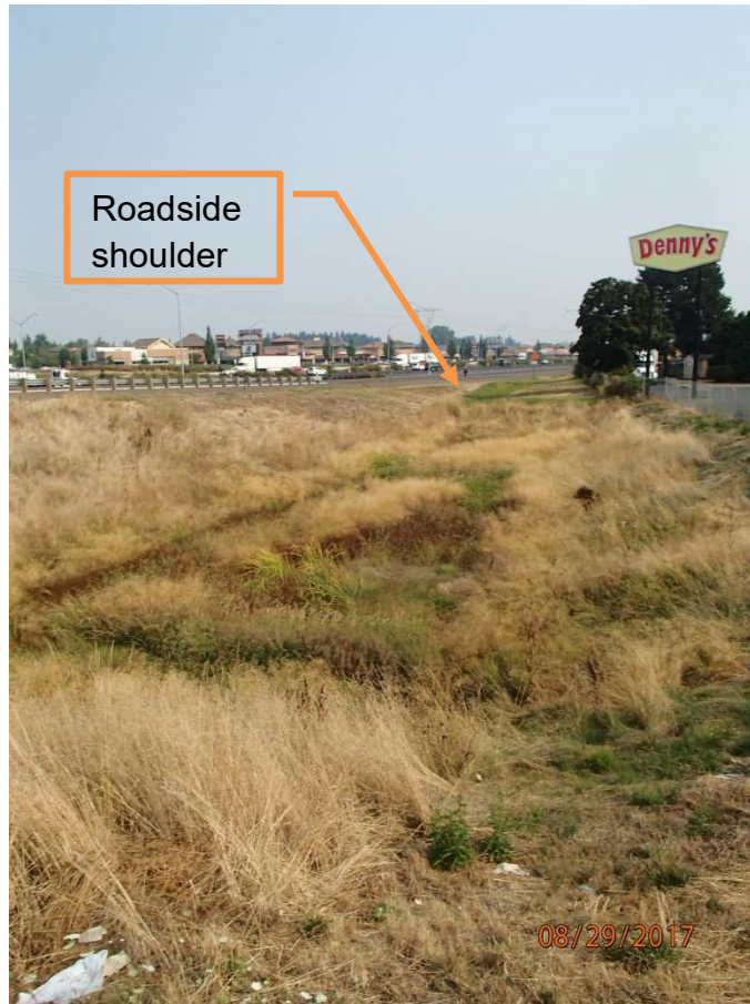
Figure 3: Roadside shoulder on I-5 ramp
