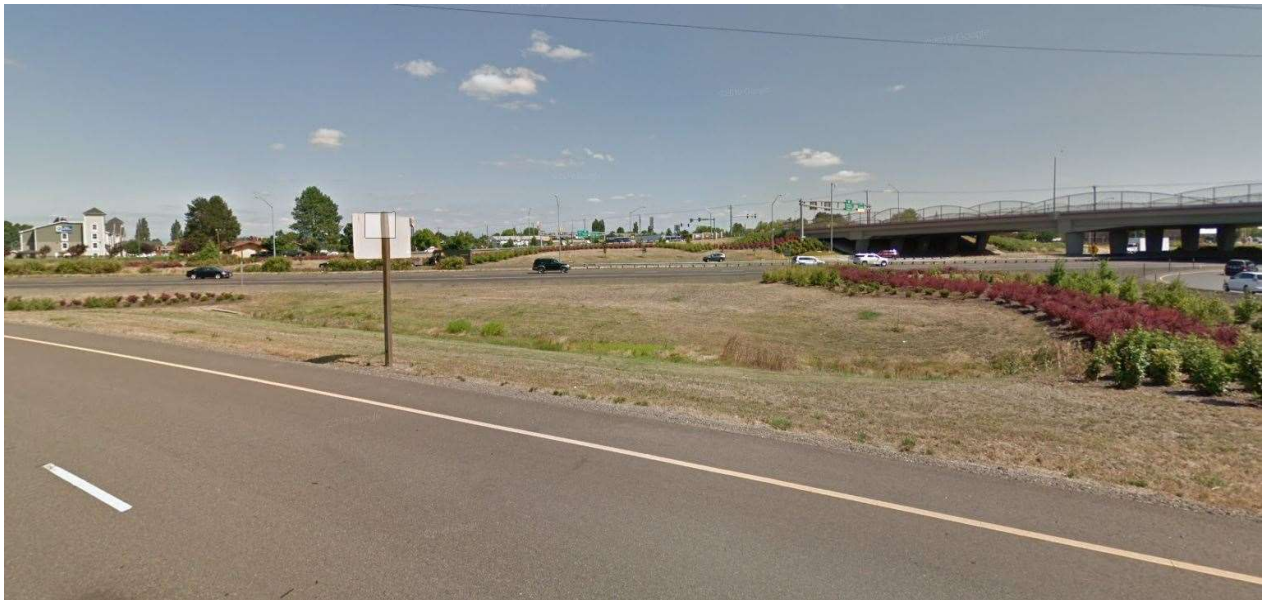
Figure 1: DFI No. D00642, (looking East on the SB off ramp)
