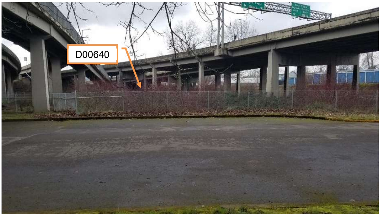
Figure 1: DFI No. D00640, looking north
