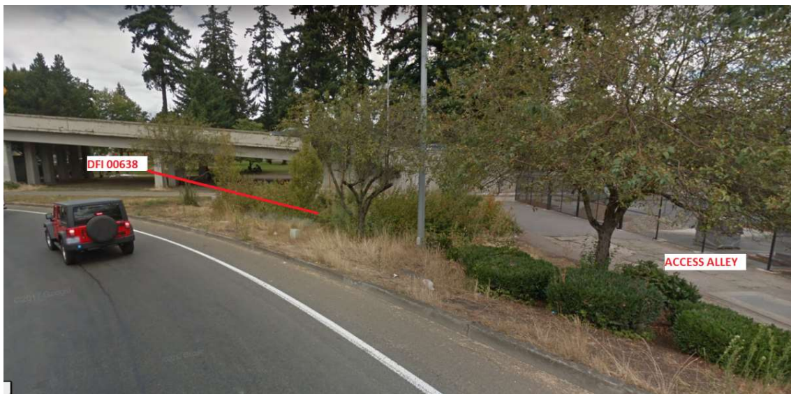
Figure 1: DFI No. D00638, looking north
