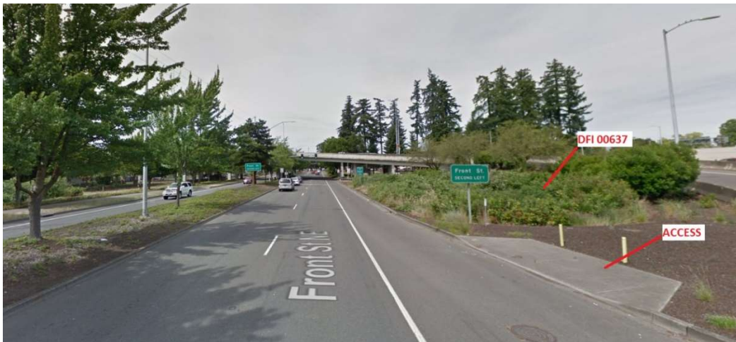
Figure 1: DFI No. D00637, looking north
