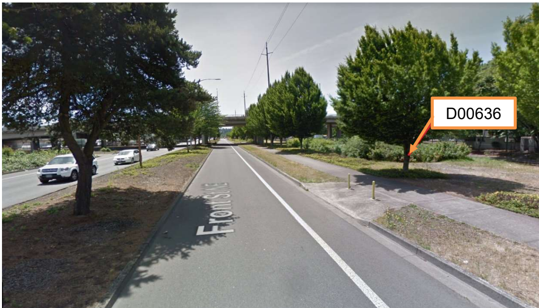
Figure 1: DFI No. D00636, looking southwest
