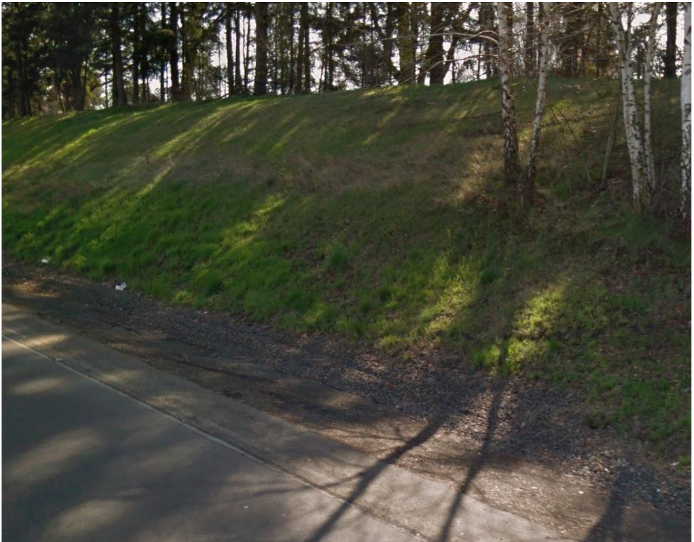
Figure 1: DFI No. D00635, looking southeast
