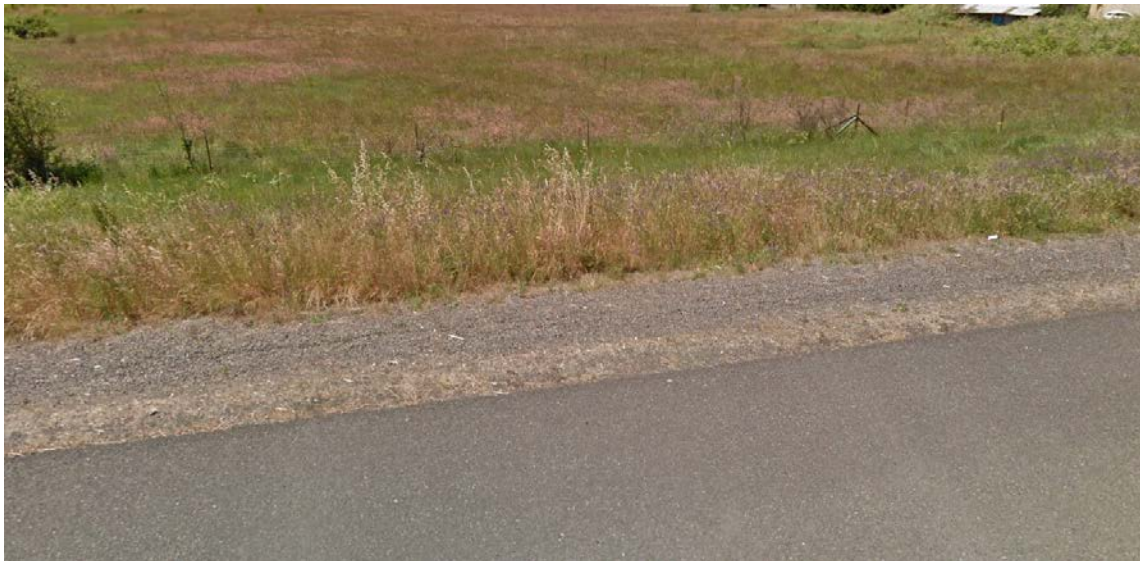
Figure 1: DFI No. D00619, looking west
