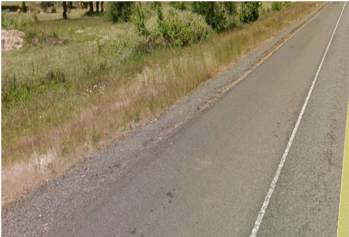
Figure 1: DFI No. D00618, looking west
