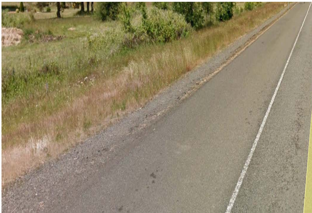
Figure 4: Facility Access along Shoulder
