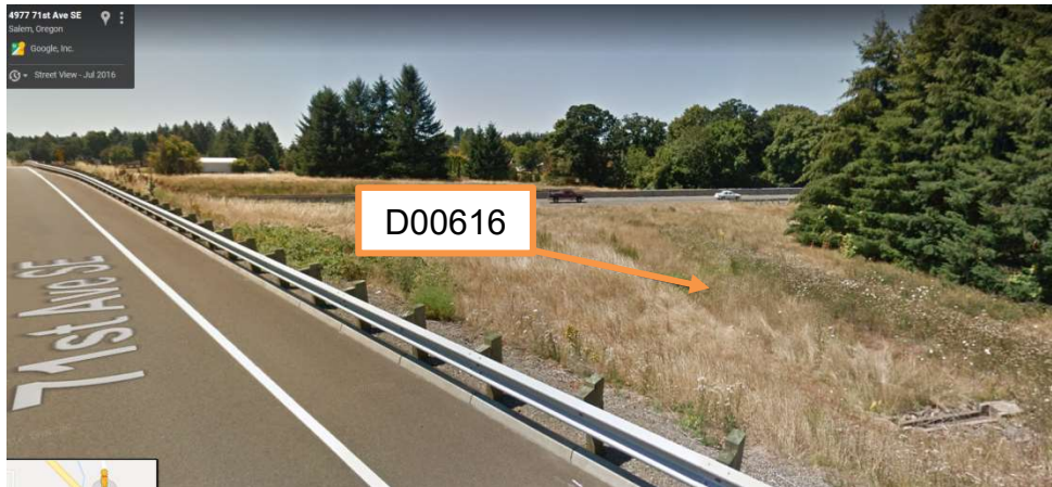
Figure 1: DFI No. D00616, looking SW from 71 st Ave overpass
