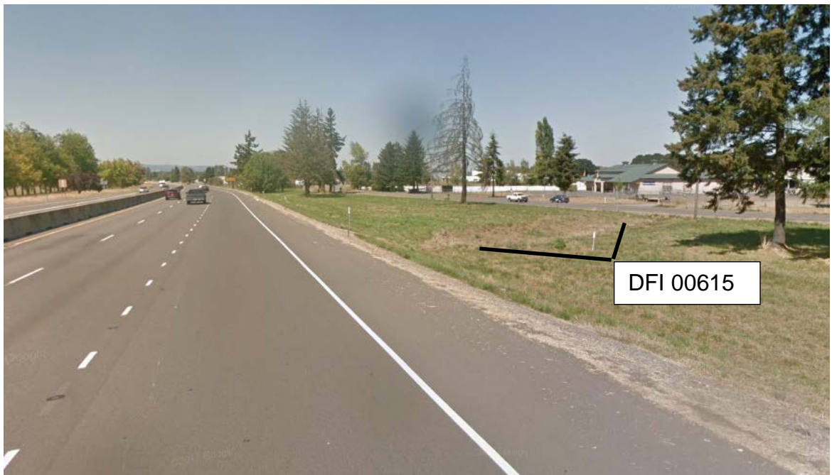
Figure 1: DFI No. D00615, looking [west]
