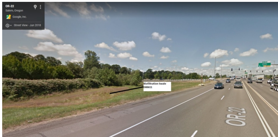
Figure 1: DFI No. D00611, looking [southwest]
