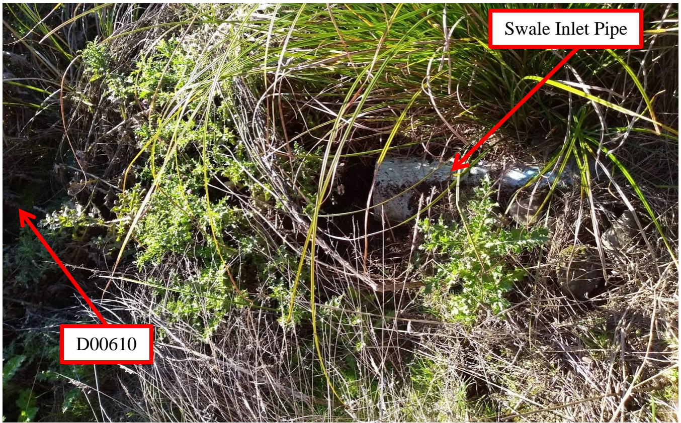
Figure 4: Swale Inlet
