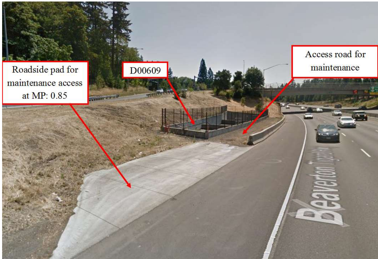
Figure 3: Access for D00609, looking south
