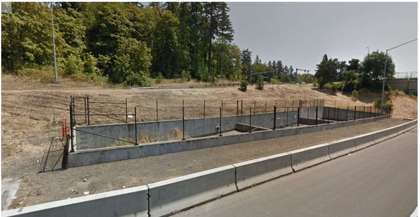
Figure 1: DFI No. D00609, looking southeast
