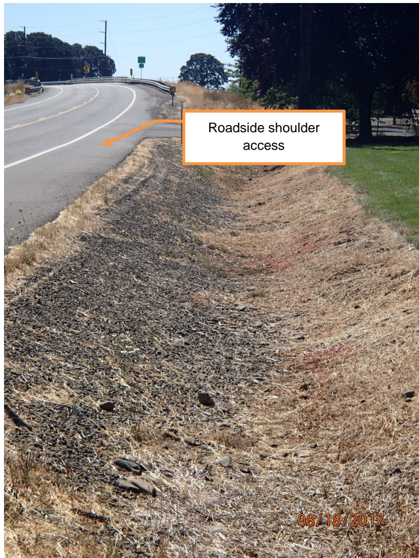
Figure 3: Swale footprint looking southwest towards Butte Creek Bridge
