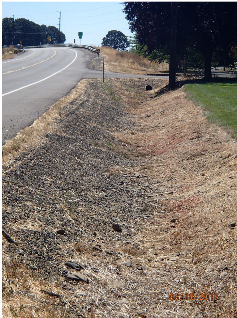
Figure 1: DFI No. D00608, looking southwest
