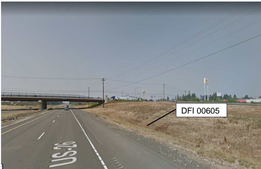
Figure 1: DFI No. D00605, looking [west]
