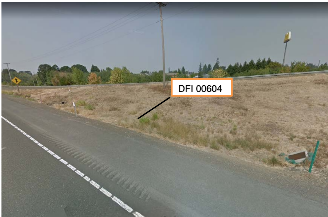
Figure 1: DFI No. D00604, looking North
