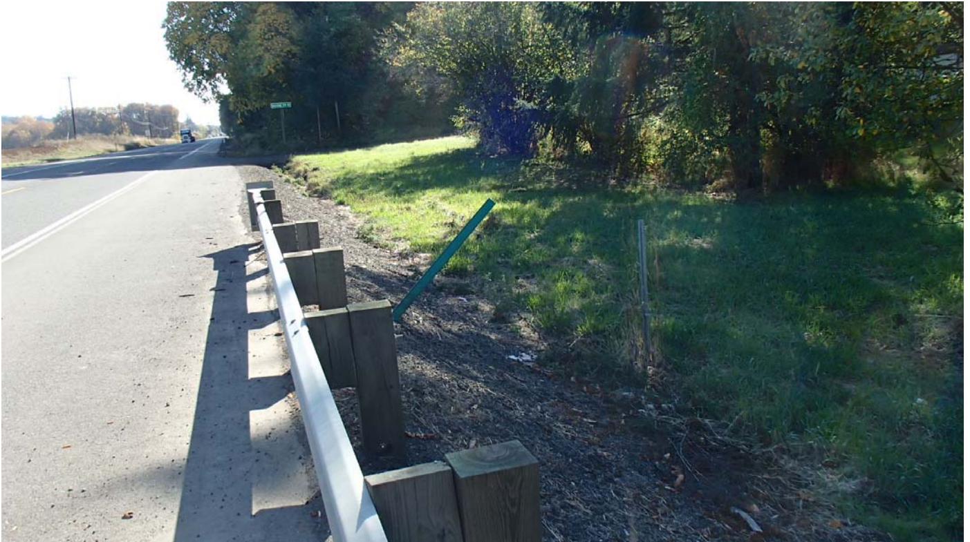
Figure 2: DFI No. D00602 looking southeast
