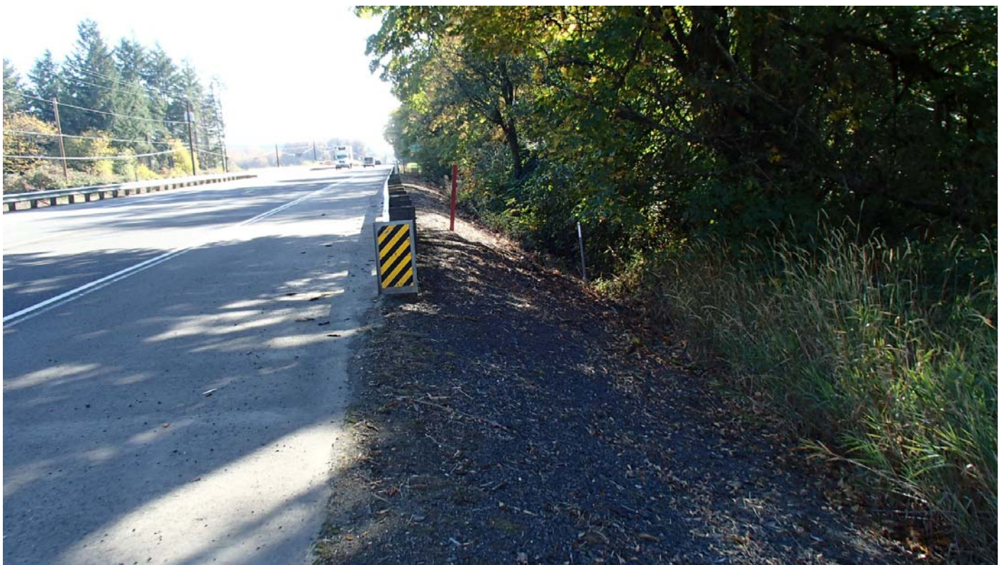
Figure 1: DFI No. D00601, looking southeast
