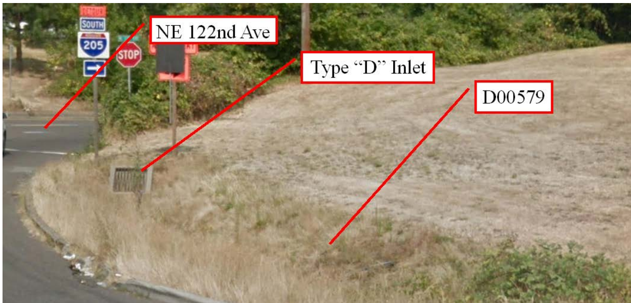
Figure 4: Swale and water inlet, looking northwest
