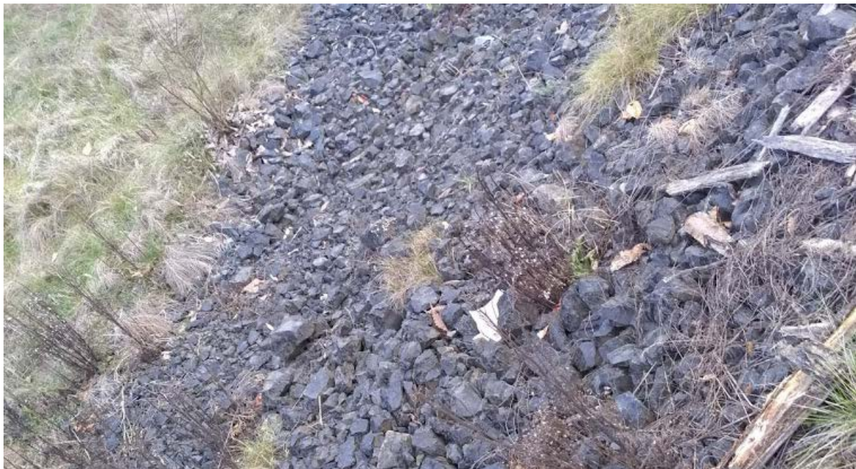
Figure 6: Granular drainage blanket
