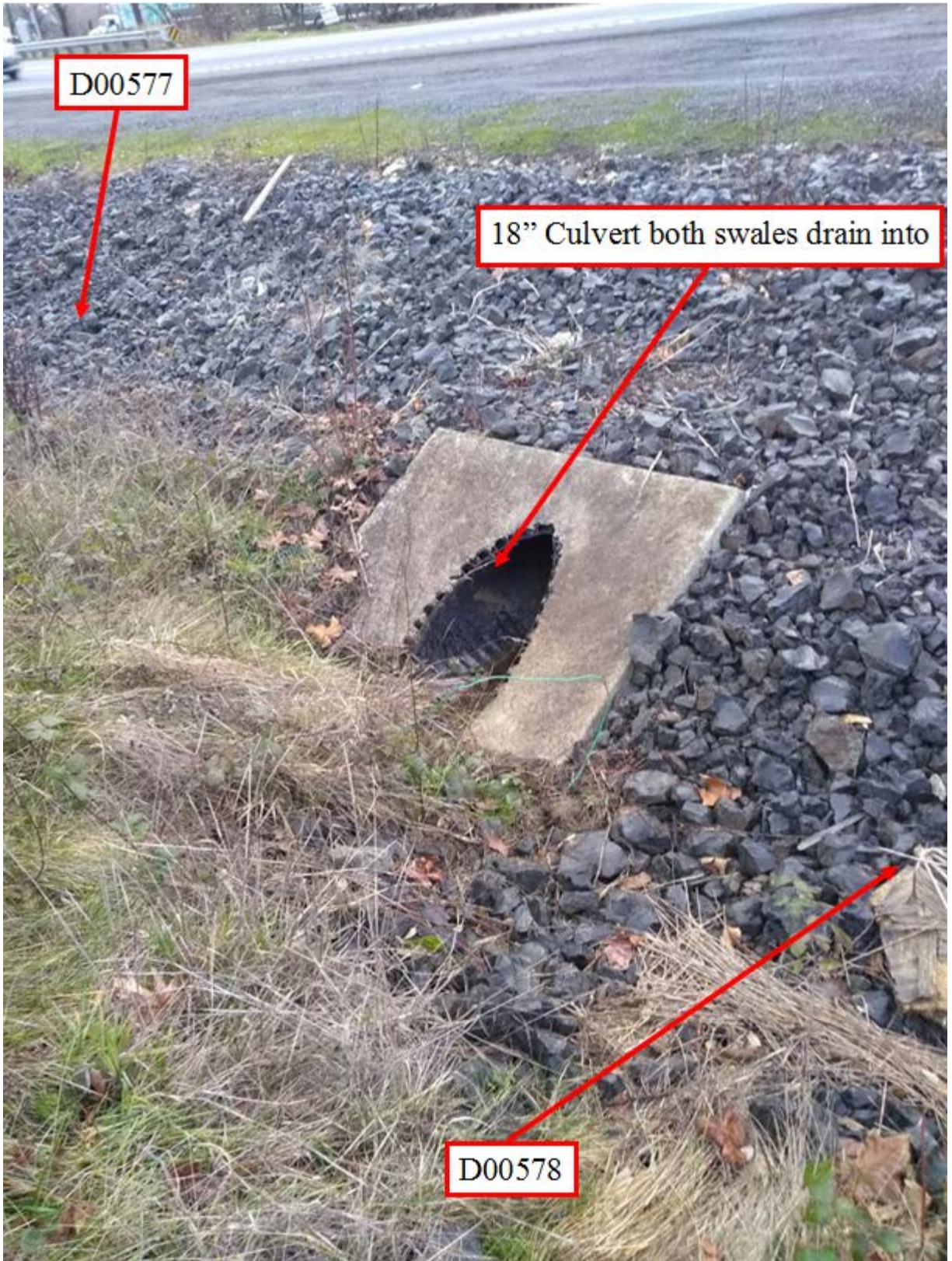
Figure 7: Drainage outlet for D00577 and D00578
