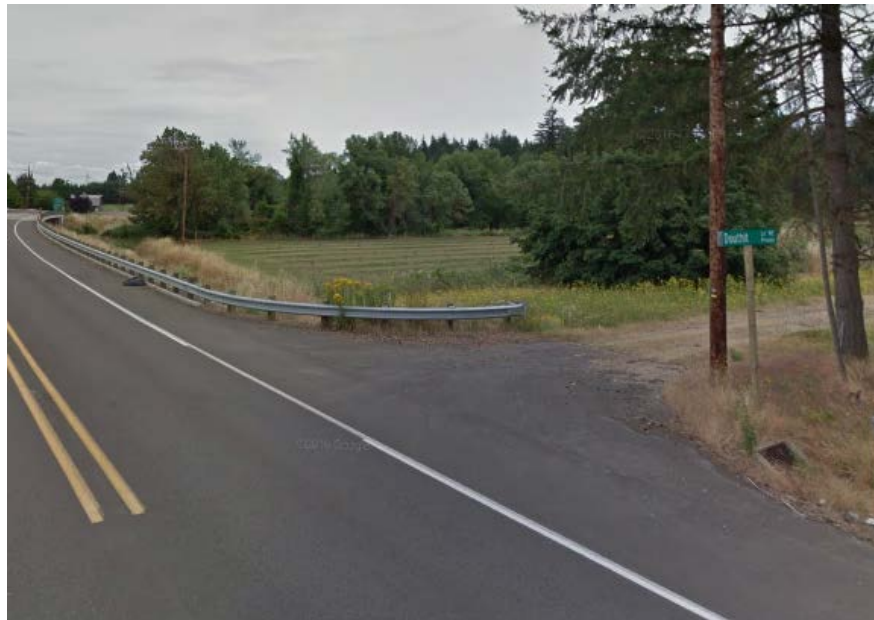
Figure 3: Facility access via Douthit Lane NE, facing east
