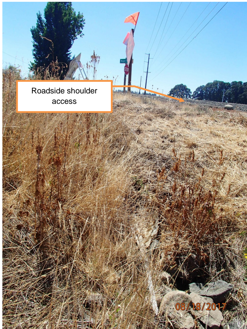
Figure 3: Swale inlet looking southwest towards Wagon Road (access)
