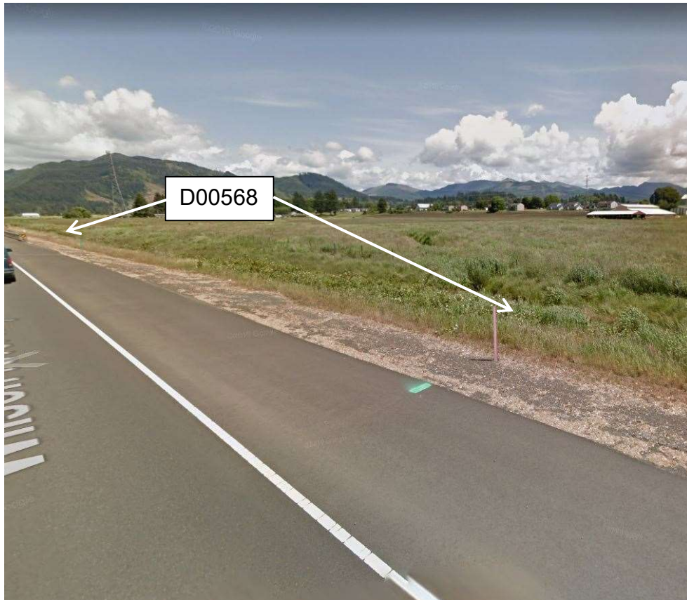
Figure 5: DFI No. D00568, looking Southeast
