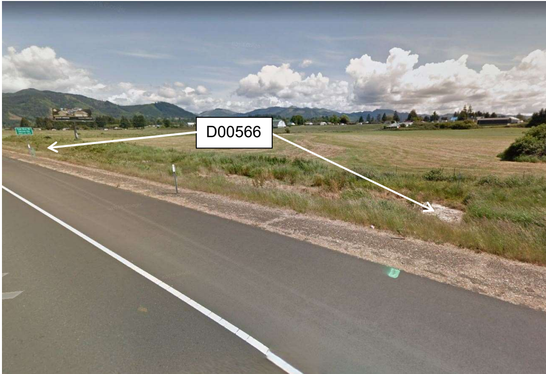
Figure 4: DFI No. D00566, looking Southeast
