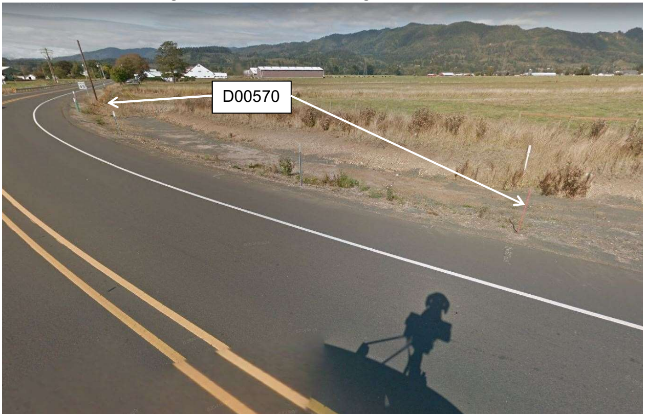
Figure 7: DFI No. D00570, looking North
