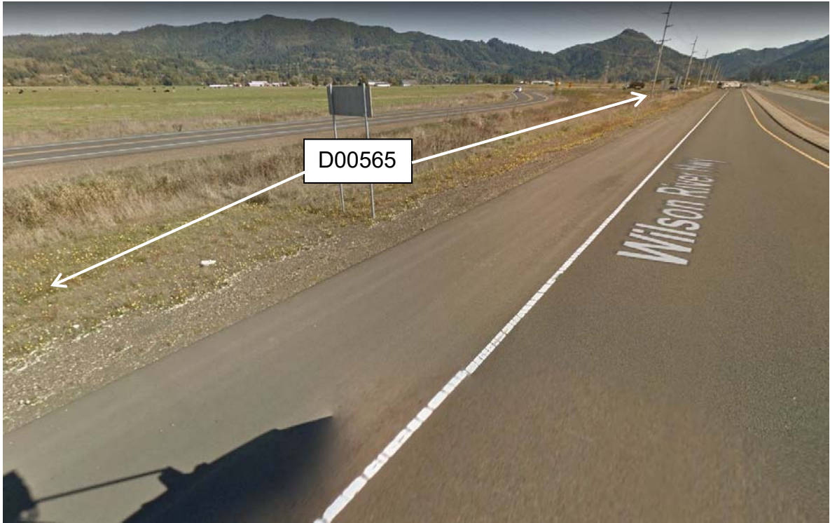
Figure 2: DFI No. D00565, looking East
