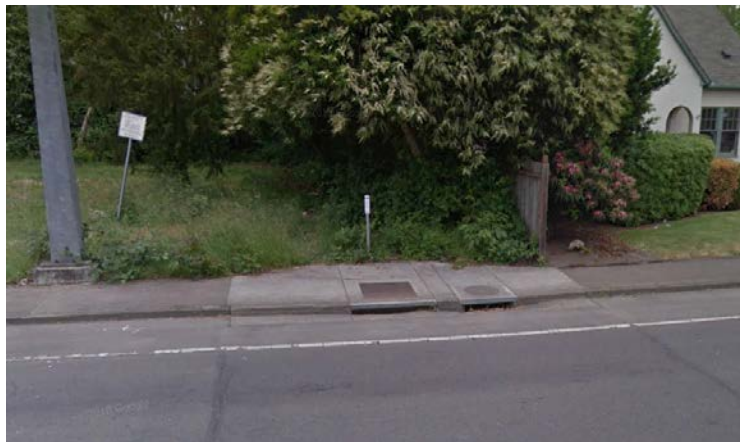
Figure 1: DFI No. D00545, looking West
