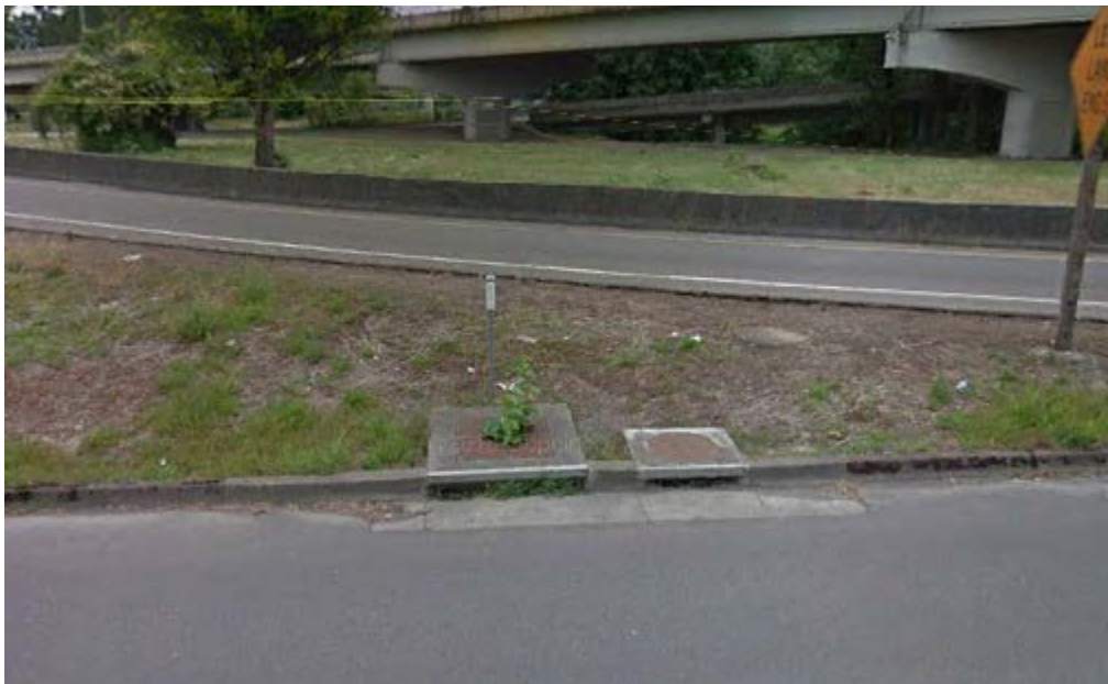
Figure 1: DFI No. D00544, looking East
