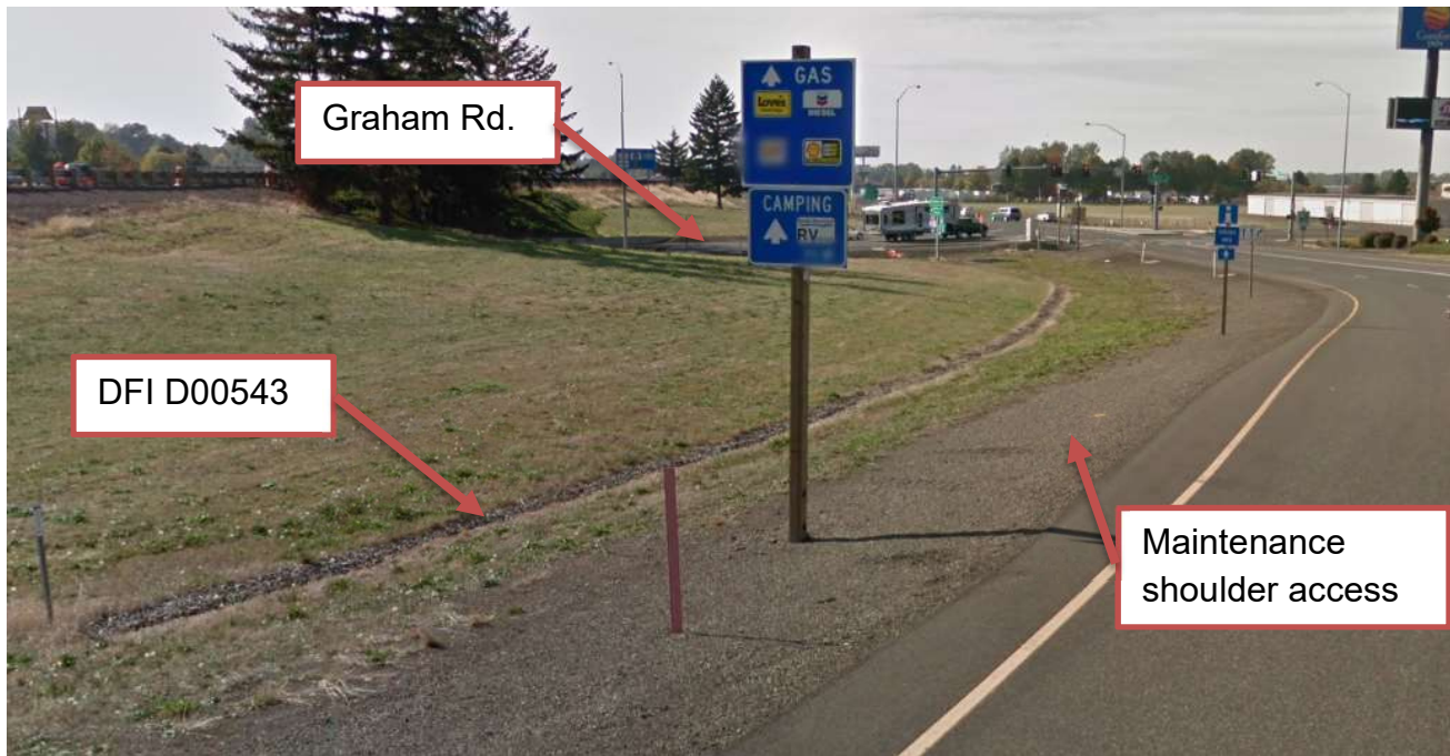
Figure 3: Looking west at Infiltration Swale
