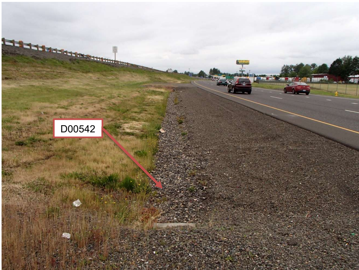
Figure 1: DFI No. D00542, looking west
