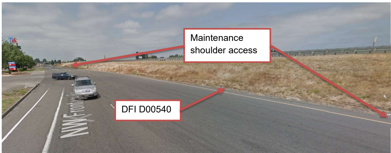
Figure 3: Looking west at Infiltration Swale
