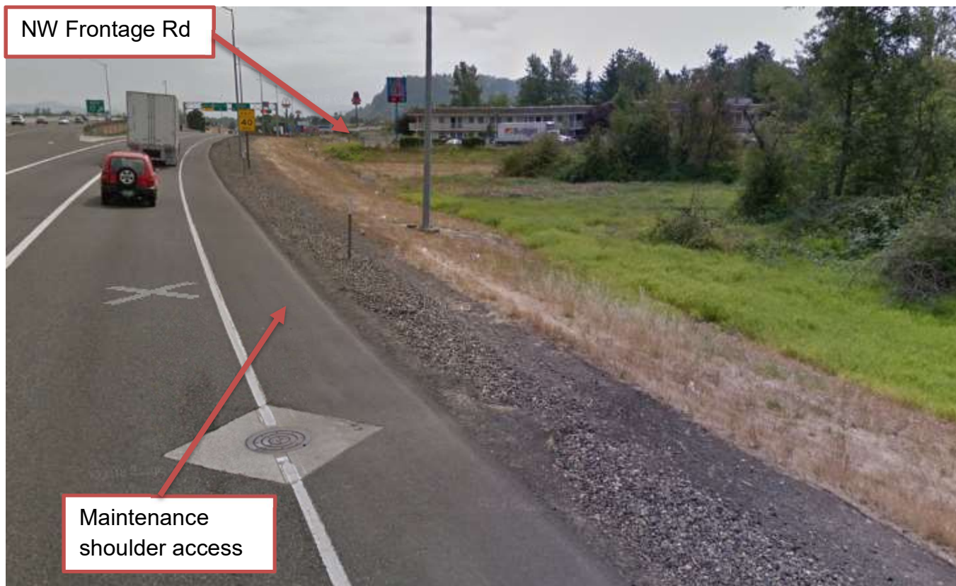
Figure 3: Looking east at Infiltration Slope
